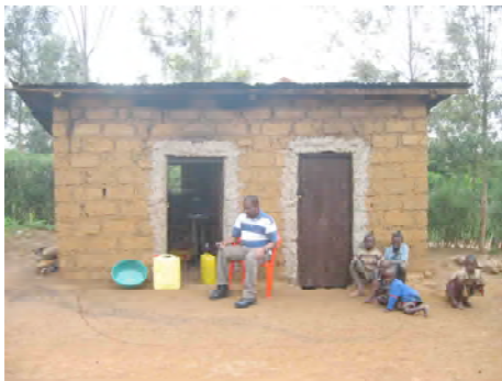
Figure 1. Test hut - left side for testing, right side for storage (new doors with locks were installed for security)
